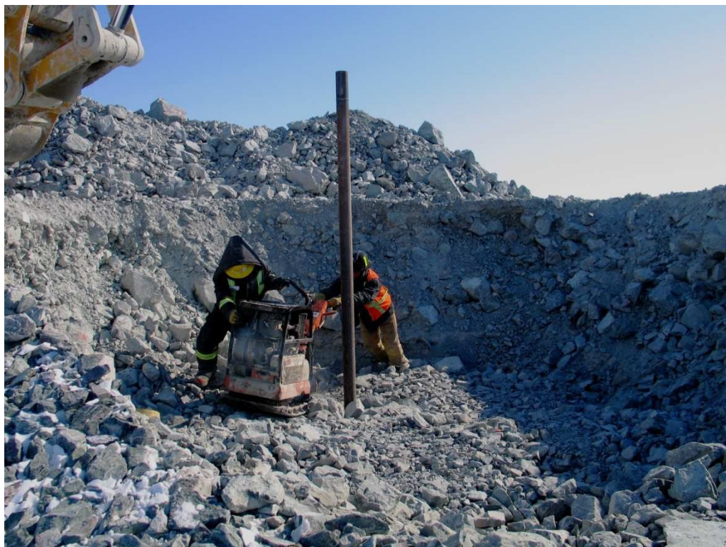
Photo 4: Hand packing first lift of ROQ at ND-SMP-080-DS
