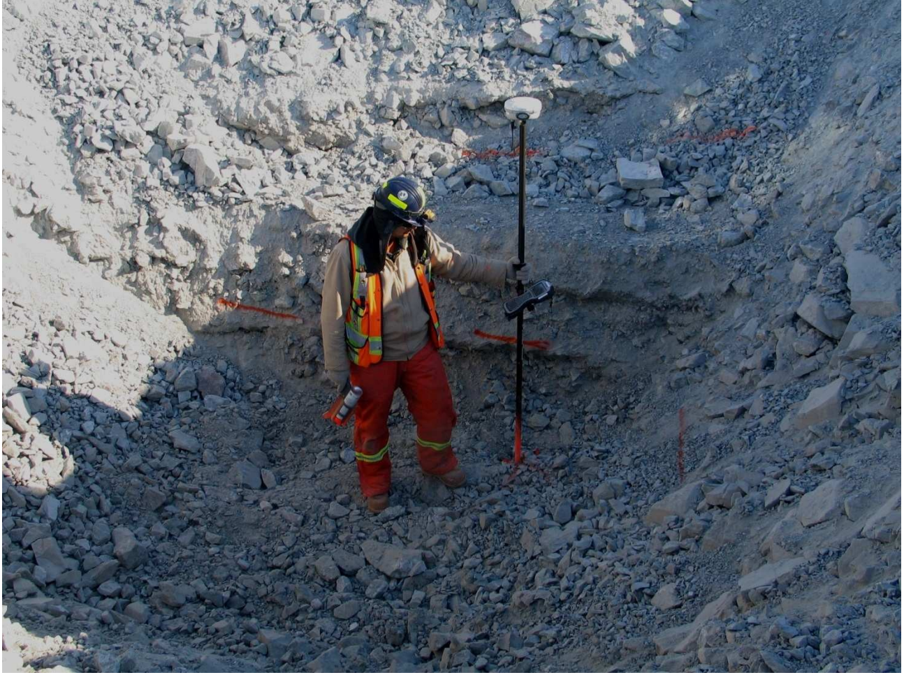
Photo 5: Excavation at ND-SMP-100-DS. Survey rod is being held at the plate center. The red line waist level of the surveyor is bottom of the plate elevation. The line above the surveyor's head is the location of the edge of the liner. The distance between the edge of the liner and the edge of the frozen core (brown in the picture) is ~ 1 meter. It is suspected that at this approximate location frozen core material was wasted as there was no where to place it. Approx..3 m of the core material was trimmed back to provide adequate width for the hand packer.
